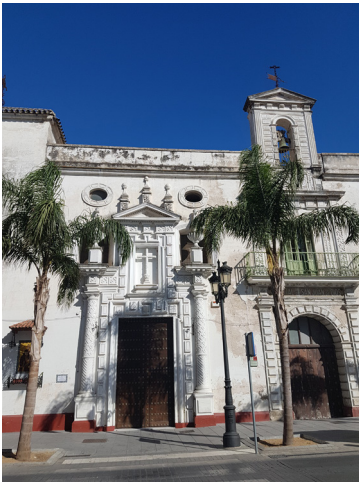
Figura 11. Hospital San Juan de Dios Fachada principal
